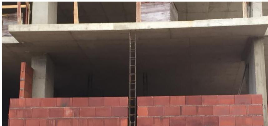
*Figure 4. An example of an intermediate column to stabilize a masonry wall (S.Brzev).*
